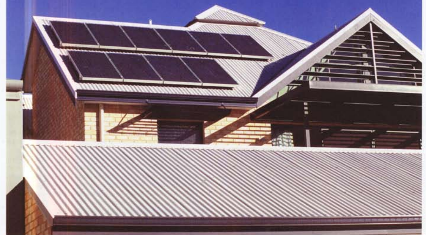
Perth's Subiaco Sustainable Demonstration Home, below and opposite page, merges sustainable design features, such as solar panels and water tanks, with visually appealing, modern construction.
